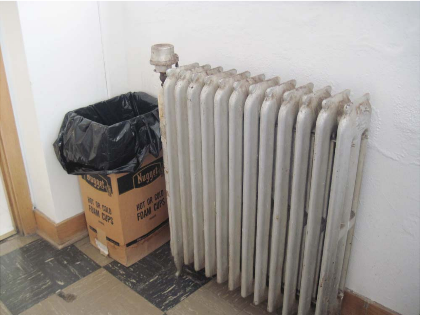
Pic #5) Recycling "bin" in breakroom placed next to radiator. Probably not an issue.
