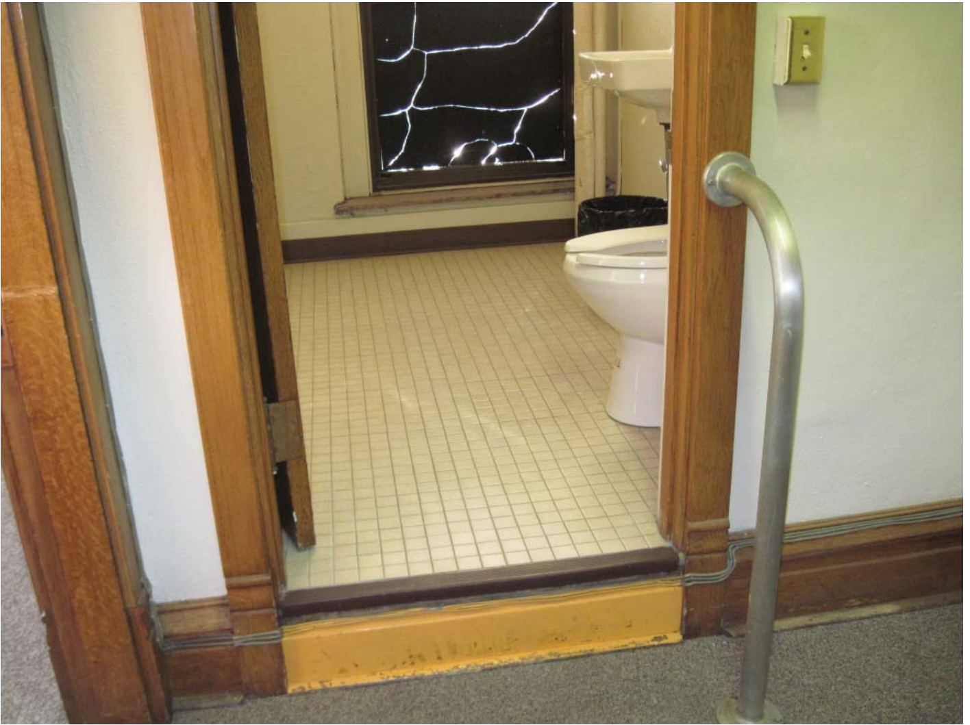
Pic #7 Restroom has painted window and step up access
