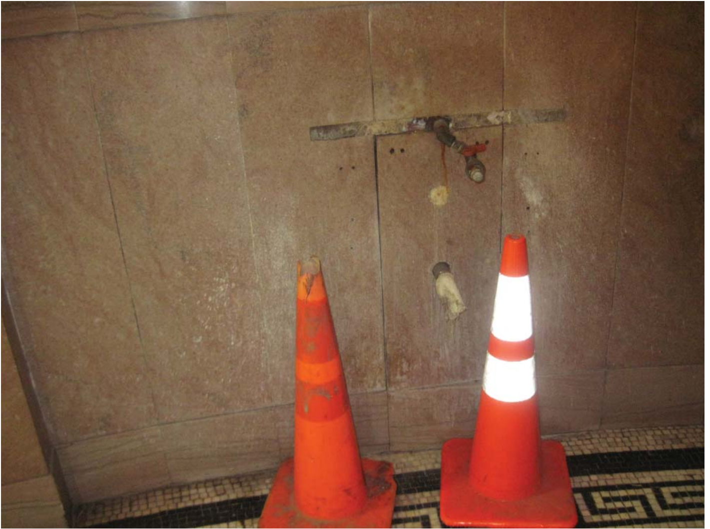
Pic #11 Repair work being done on drinking fountain issue.
