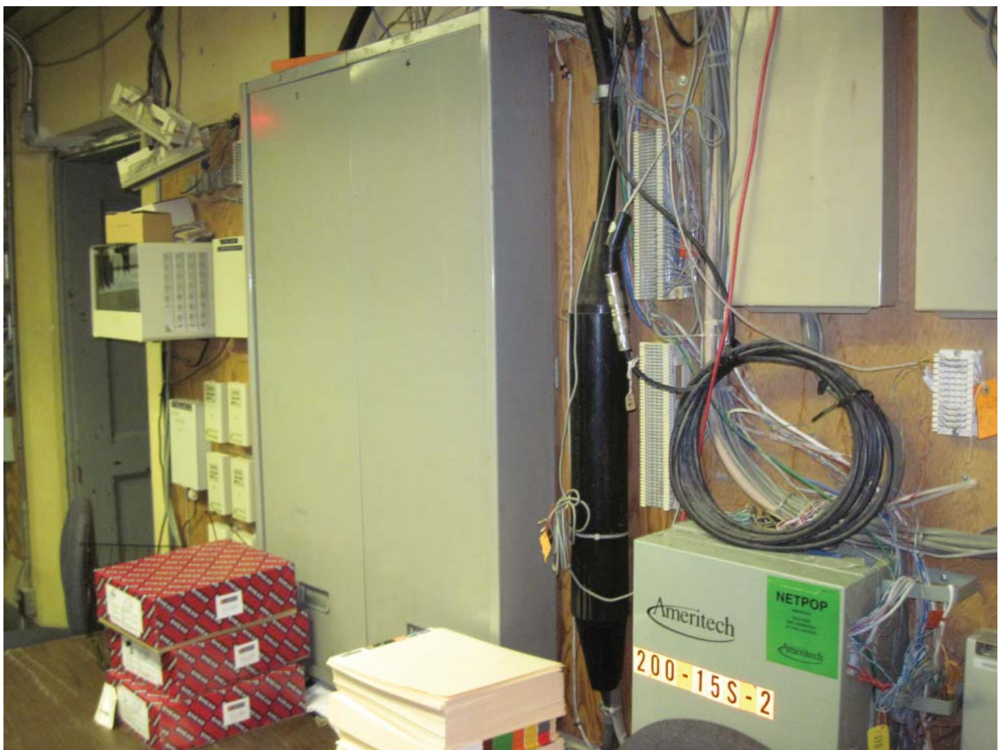
Pic #14 Storage area in basement
