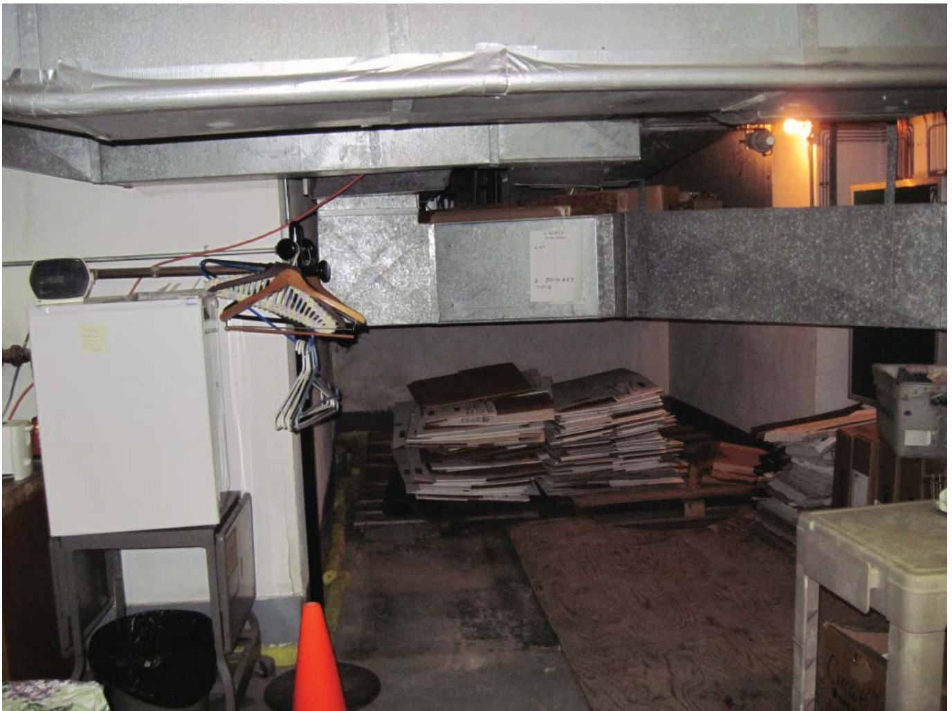
Pic #13 Storage area in basement
